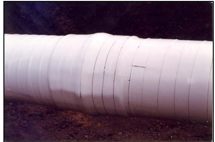
600 Series Coating applied on a rehabilitation project.
